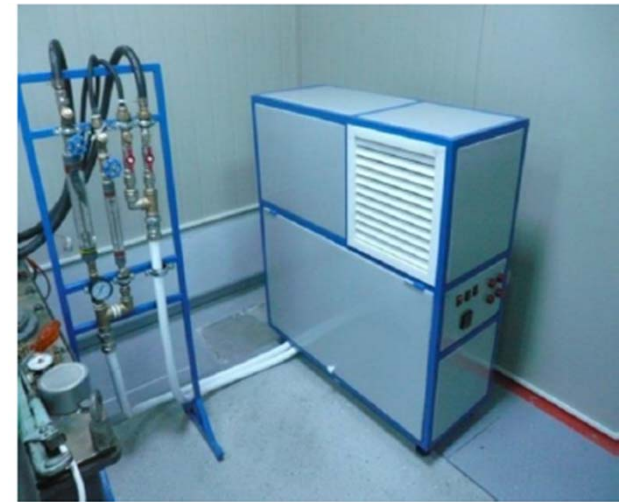
Klystron Thermoregulation System
