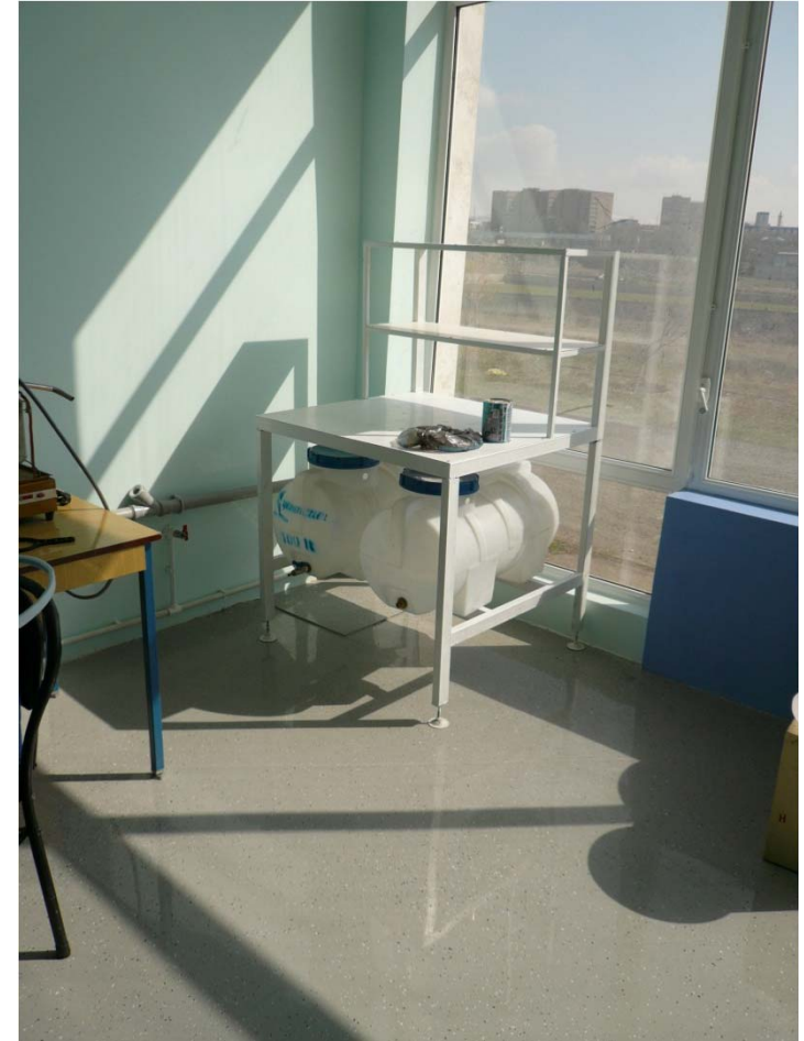
Water storage tanks
