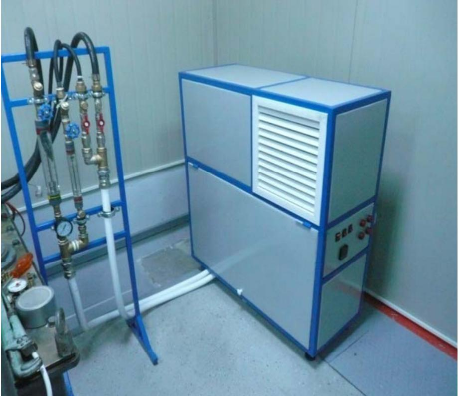
Real Cooling System of Klystron
