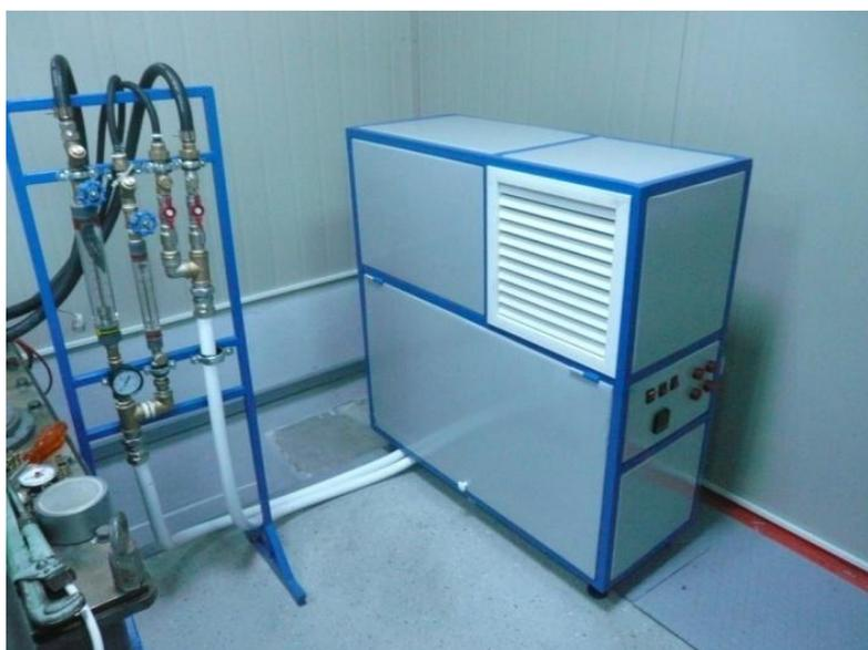
Figure 1.5.3.2.: Realistic view of klystron's thermoregulation system.
