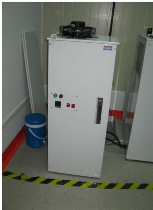
Figure 1.5.2.2: Thermoregulation system for RF gun.
